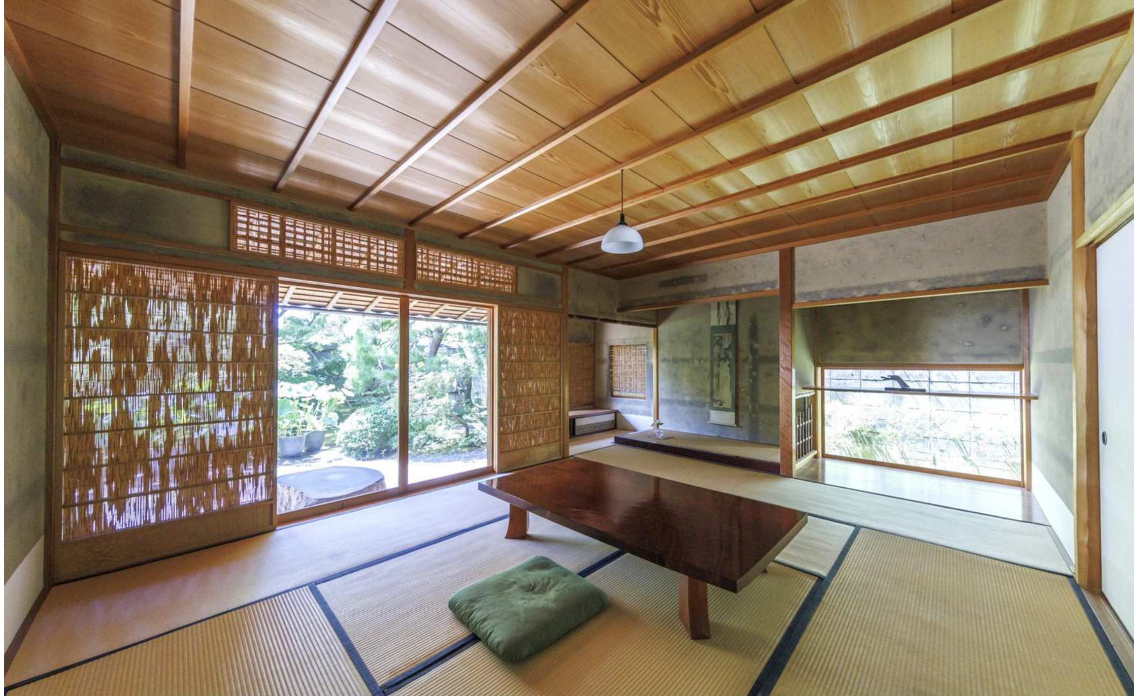
A tatami room of 10 jo (1 jo = 1.62 m 2 ) with "Deshoin (Samurai-residence style attached towards an alcove. Paper sliding doors are replaced by bamboo doors. Pillars are chamfered columns made by shaving the four surfaces of Kitayama Maruta to show grains. A big eave supported by small-diameter Kitayama Maruta sticks out into the garden, connecting the building and the garden.
